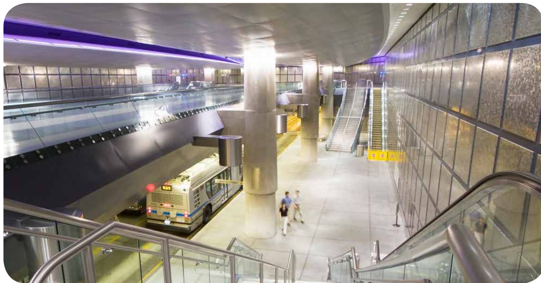
Enclosed BRT Station and Transfer Area
